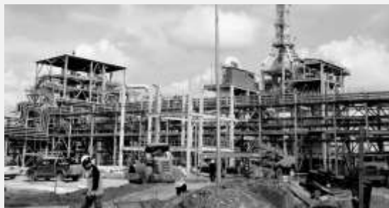
Lynas factory in Kuantan during construction.
